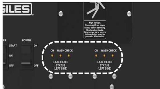
**[WASH]** light is **NOT** intended as the signal for routine cleaning of the cell, **DO NOT use it as such**. Typically, the collection cell must be cleaned **DAILY** to ensure optimum performance. See [Section 4.04.2, EAC Filter Cell Cleaning](#).
